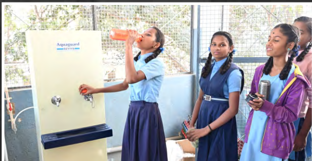
RO water filters have been distributed in all schools, and plumbing and electrical installations have been identified for implementation
