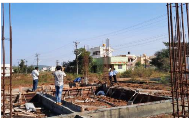
Dharwad Building construction
